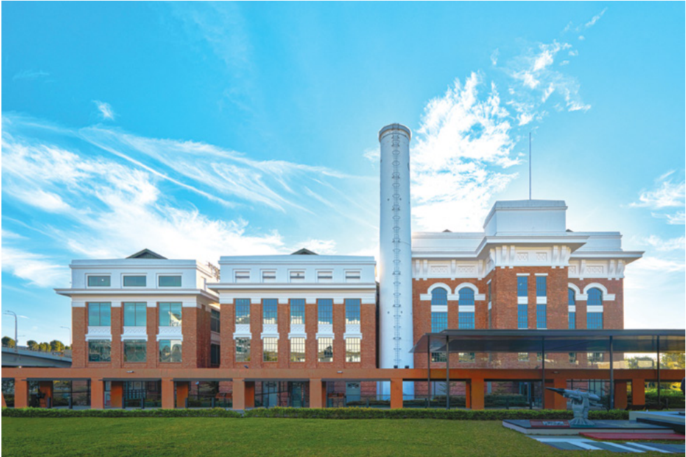
The St James Power Station today, after it was redeveloped and gazetted as a national monument. Source: Mapletree Investments Pte Ltd
